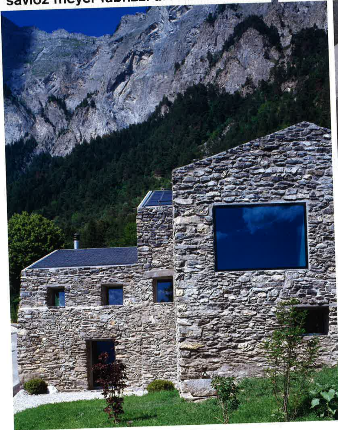
Roduit House, Chamoson, Switzerland, 2004-5. The original building, constructed in stages since 1814, is made up of three adjacent volumes on different levels. The old stone construction echoes the rocky mountainside, and the renovation project sought to maintain and reinforce this character, while using concrete for the interior renovation. The exterior volume was not changed; the stone facades were preserved and lined with an insulating layer of concrete based on foamed recycled glass (Misapor).
